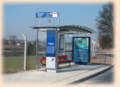
High-tech Fastrack stop and information point.
